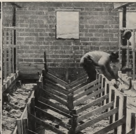
Forming in place for mangers.
